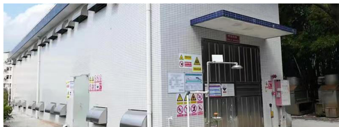
In our China facility, we store hazardous chemicals separately at the Class A warehouse, which was built in line with the Code for Fire Protection Design of Building, aiming to guarantee the safety of the chemicals
