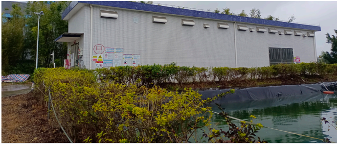
The warehouse was divided into four separate areas to fulfill different chemical storage requirements
