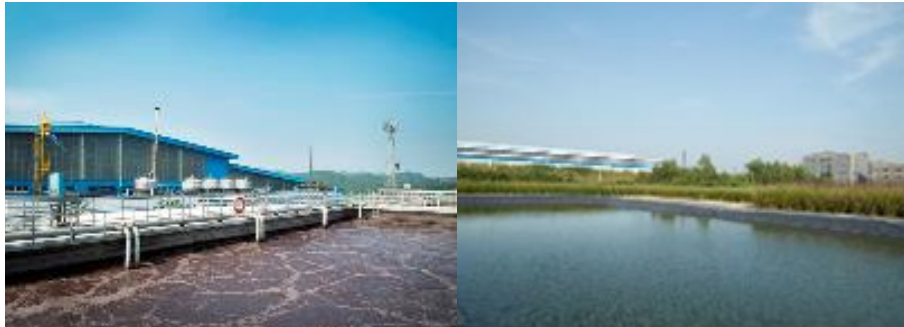
WWTP and Wetlands of China facility
