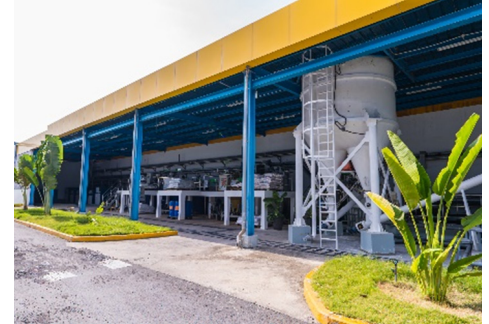
WWTP of Vietnam facility
