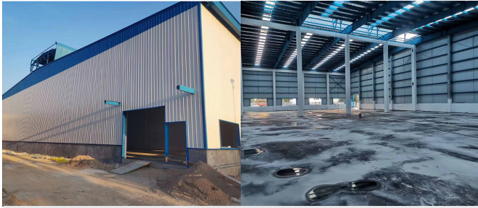
Brand new Class C chemical warehouse in China
